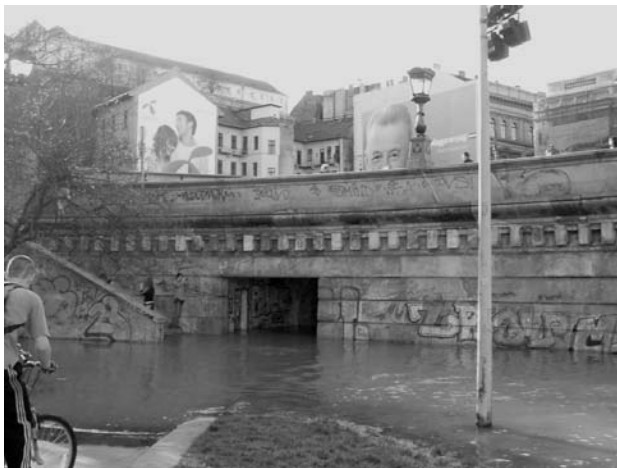
Flooded tunnel in Budapest
